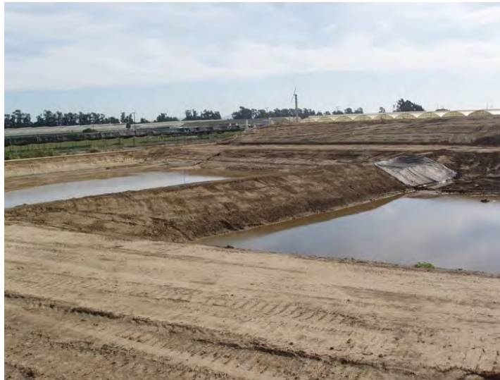
Fig. 1. Impoundments such as detention basins capture runoff water so that it remains on the nursery site. This helps to prevent the movement of pollutants into water bodies. Photo by Julie Newman.
