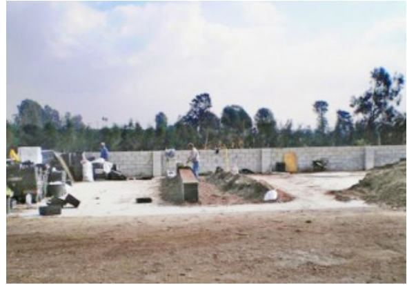
Fig. 1. A concrete storage pad and retaining wall are used to store and mix media with fertilizers. This reduces the movement of soil particles and fertilizers. Photo: D. Zurawski and J.P. Newman.
