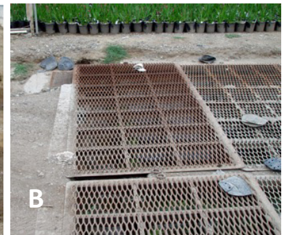
Fig. 5. Shallow sediment trap used by a small nursery to remove large, heavy particles such as sand. Sediment trap shown without the cover (A) and with a grate so vehicles can drive over it (B).
