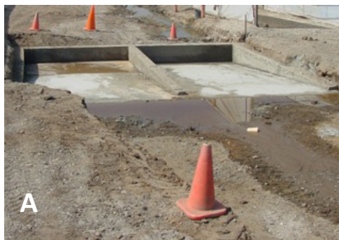
Fig. 5. Shallow sediment trap used by a small nursery to remove large, heavy particles such as sand. Sediment trap shown without the cover (A) and with a grate so vehicles can drive over it (B).
