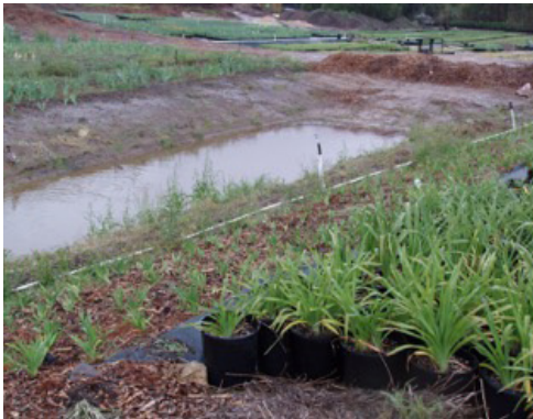
Fig. 6. A sediment basin temporarily detains sediment-laden runoff under quiescent conditions, allowing sediment to settle out. Photo: J.P. Newman.
