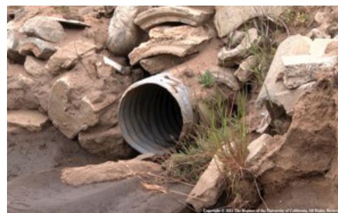
Fig. 3. Corrugated metal culvert drain pipe. Culverts provide cross drainage for roads with inside ditches. Photo: R. Lucas.
