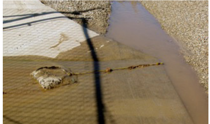
Fig. 12. Polyacrylamide (PAM), a flocculant held in the anchored bag, removes sediment from runoff entering a retention basin. Photo: A. Storm and J.P. Newman.
