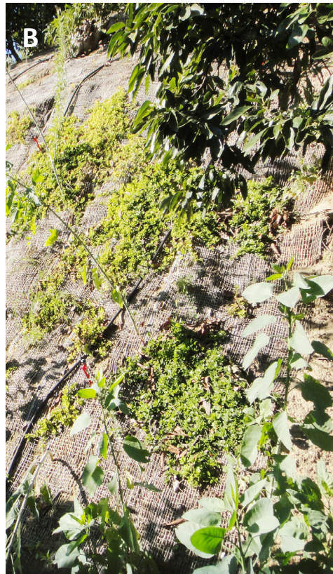
Fig. 4. Controlling hillside erosion. A critical area planting (A), comprised of a mix of ornamental species planted on this roadside hill, is being used to improve slope stability; the roots anchor the soil and trap runoff, resulting in reduced sediment loads. Jute mesh (B) is being used to retain soil on the slope while plants are becoming established. The netting is biodegradable and turns into organic matter in the soil. Photos: S. Webb, courtesy of the Resource Conservation District, Ventura County.
