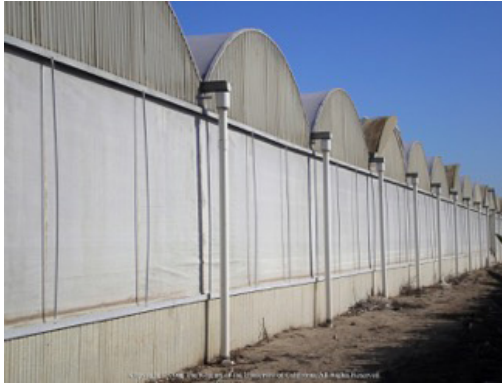
Fig. 10. Rainwater in this nursery is collected and piped underground to a retention basin. Photo: D. Zurawski and J.P. Newman.
