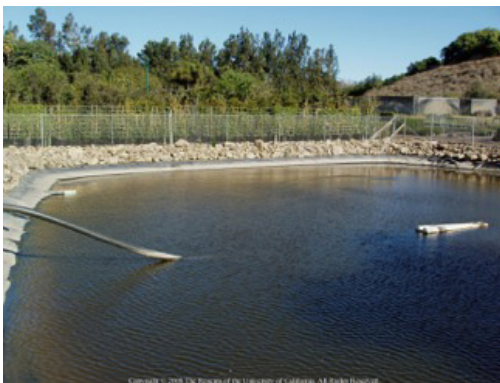
Fig. 11. This lined retention basin has rock rip-rap along the sides for stabilization. Photo: D. Zurawski and J.P. Newman.
