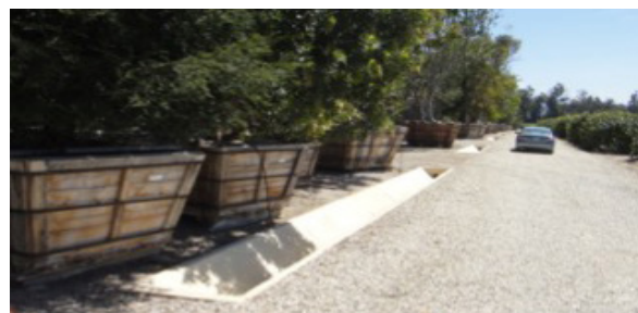
Fig. 2. Concrete V-ditches prevent runoff water from picking up sediment and carrying it downstream. Gravel access ways increase surface area for water to impact and absorb into the soil. The gravel stays on the surface of the soil allowing for traffic in wet weather, and soil is not moved by runoff or vehicular traffic. Photo: S. Webb, courtesy of the Resource Conservation District, Ventura County.
