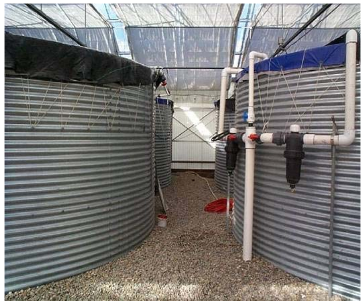
Fig. 1. Before water is re-used on greenhouse crops in this nursery, it is heat-treated to reduce pathogens. These tanks store the heat-treated recycled water. Photo: J. Newman.
